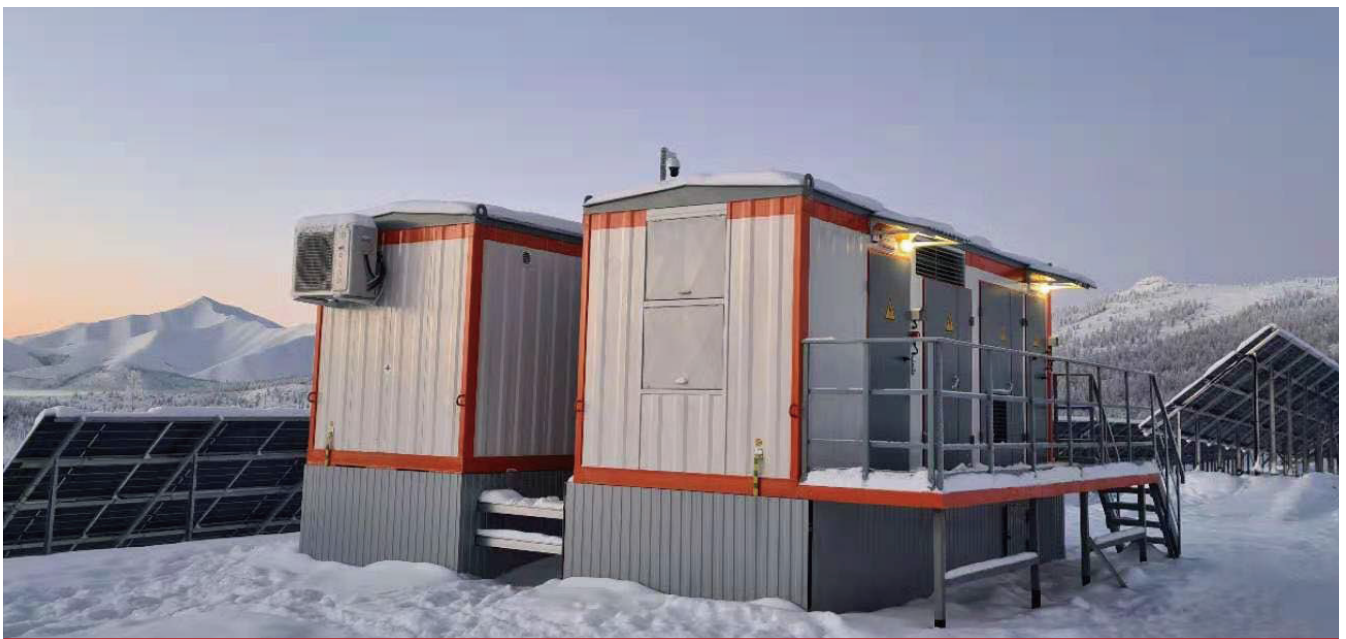
1 MW Energy Storage Project in Europe
